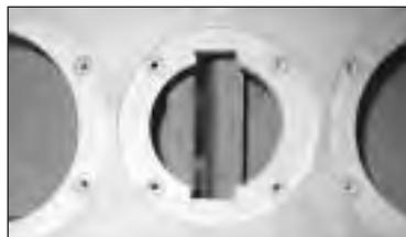
**PHOTO 6:** Threaded brass inserts were used for mounting the drivers.
