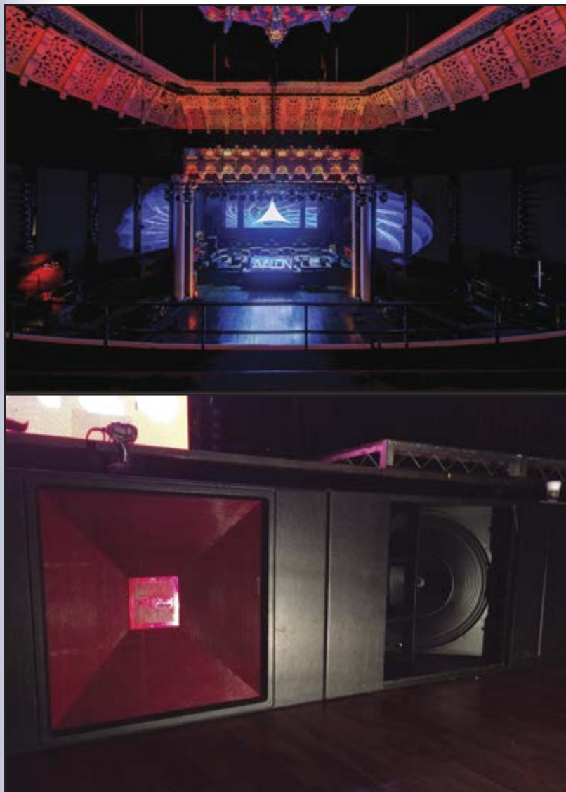
The Avalon Hollywood club now has a new improved audio system, featuring “the world’s largest subwoofer club installation ever” with new subwoofers powered by Powersoft’s new M-Force technology and 40” cones.
